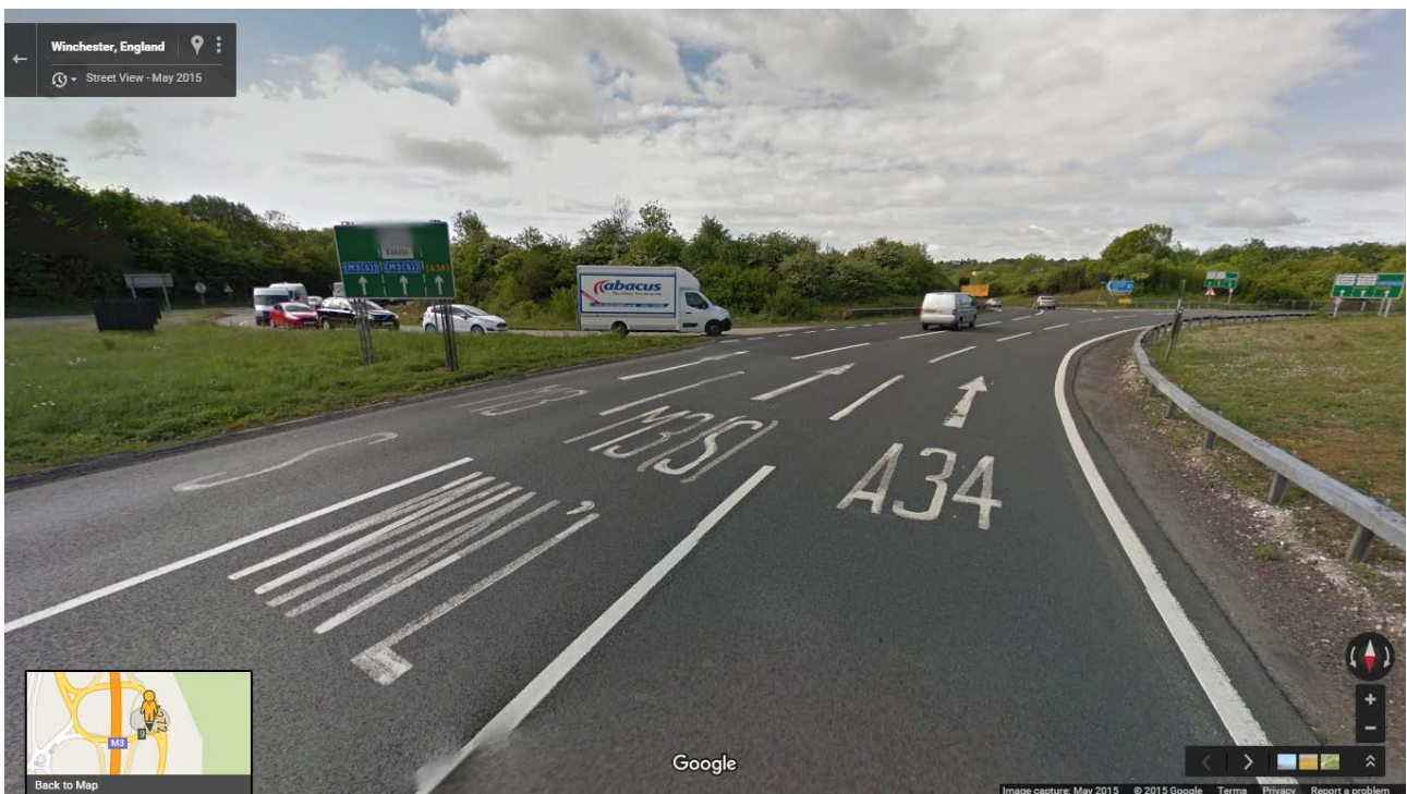
Above: Eastern circulatory carriageway widened to three lanes © Google 2015
